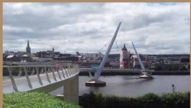
The new Regional Policy provides support for projects such as the Peace Bridge in Derry, Northern Ireland.
