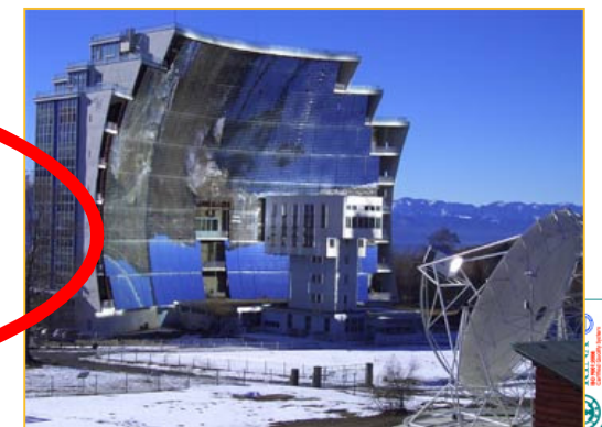
PROMES-CNRS solar plant
